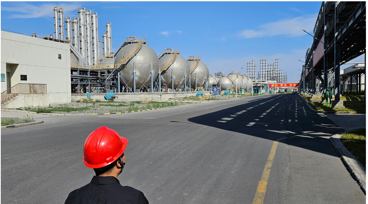
Xinjiang province, China. Site tours of Daqo New Energy's factories in the region. The large spherical tanks contain hydrochloric acid, while the cylindrical towers are used for distillation, both needed for the production of polysilicon which is the most important material used in solar modules.
